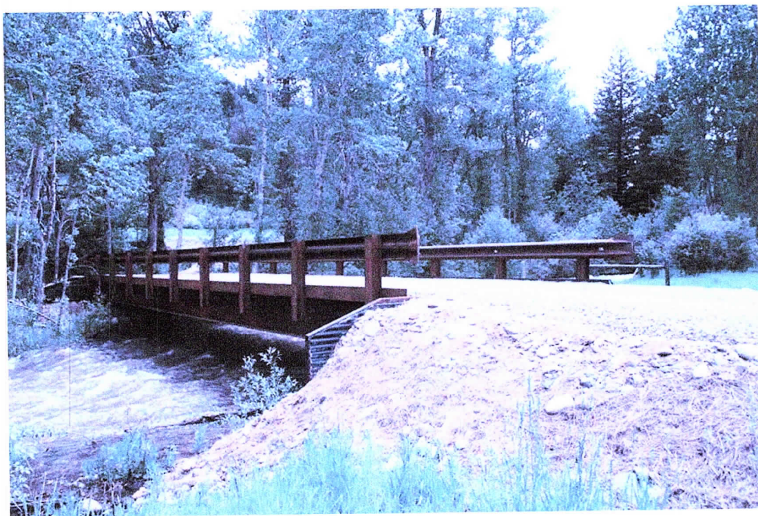
16' x 65' TNS Mod Bridge. Please note the steel backwall on the end of the bridge
